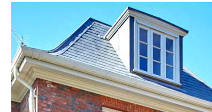
EXAMPLE OF PROPOSED LEAD DORMER TO REAR ELEVATION (LOWER WINGS)
